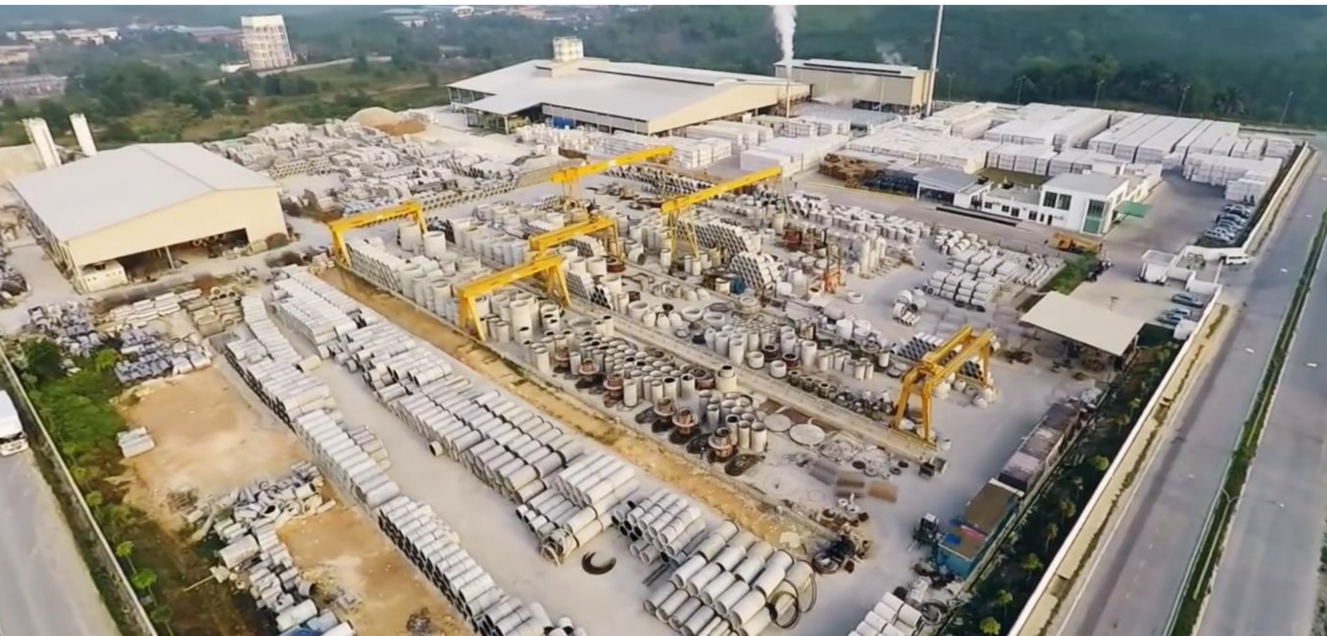
G-Cast Precast Concrete Factory @ Serendah
